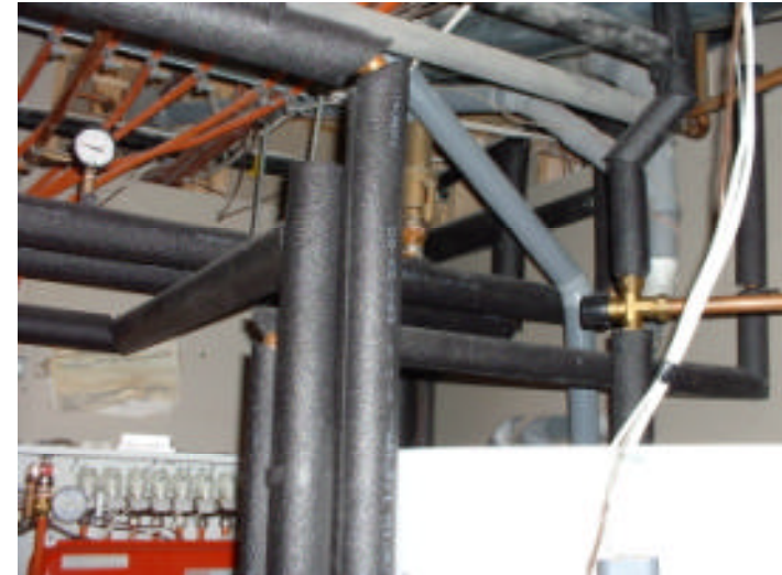
^ The copper tubing in the middle (covered with foam insulation) is the feed from the solar hot water panels on the roof. These supply heated liquid to the storage tank.
